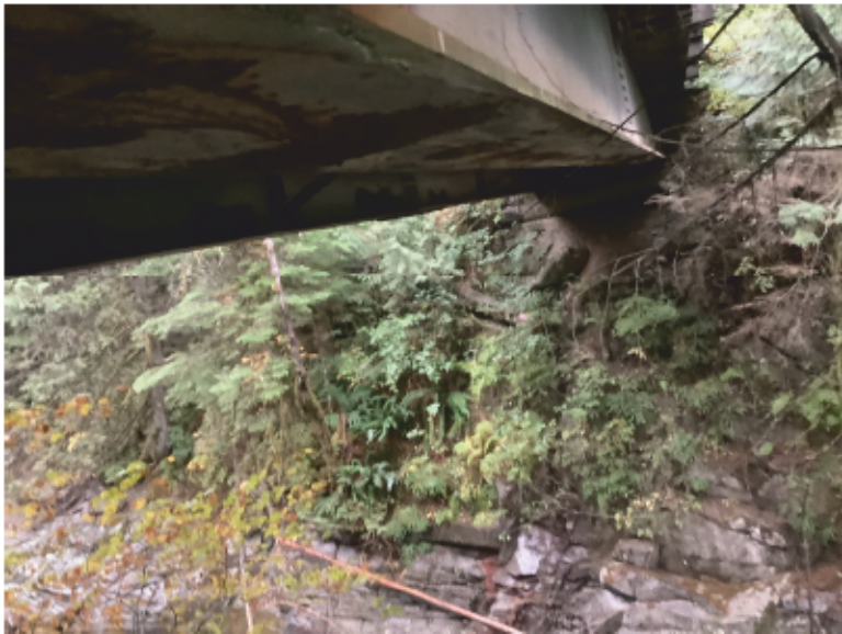
Left Bank Abutment when facing downstream
