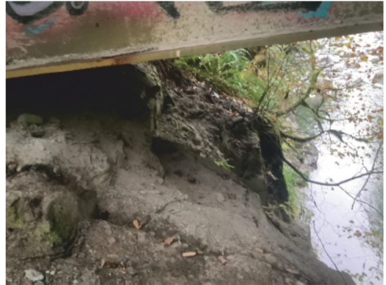
Right Bank Abutment when facing downstream
