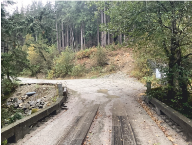
Approach from bridge deck of Right bank approach when facing downstream
